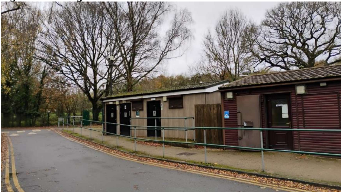
Figure 9: Existing Willow Lawn toilet block.
