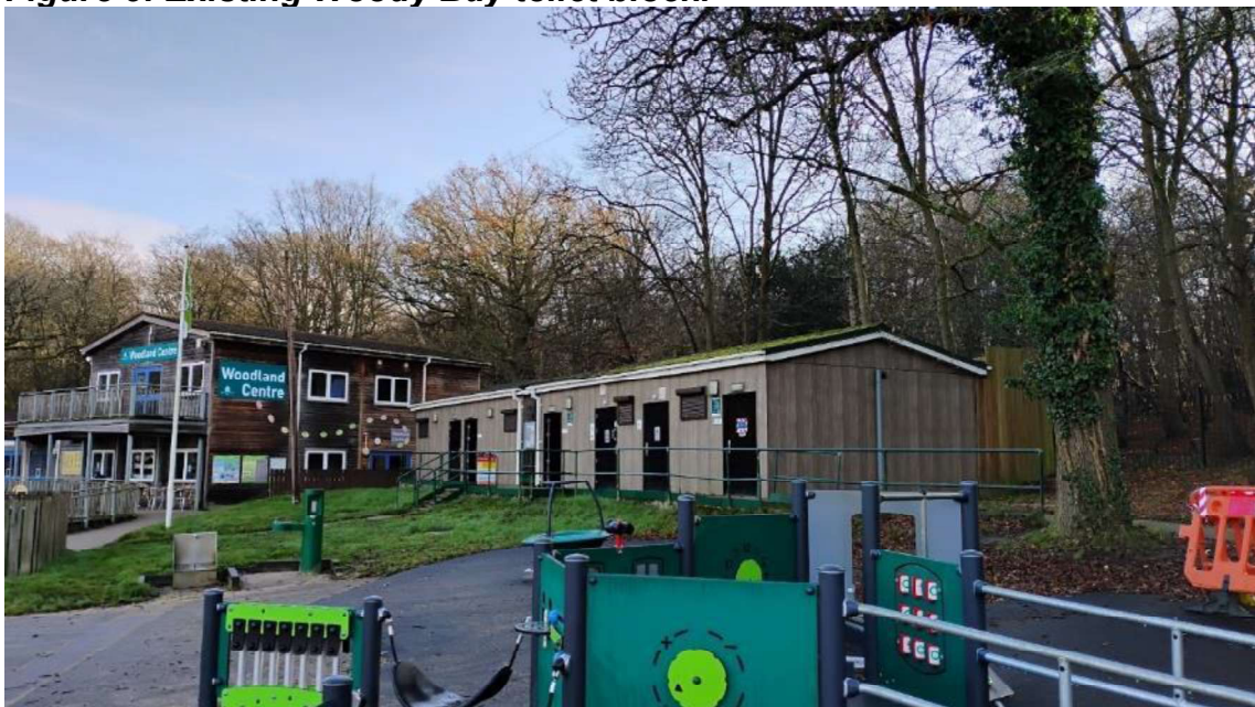
Figure 5: Existing Woody Bay toilet block.
